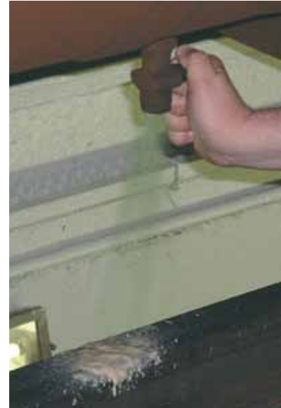
Mayonnaise removed from an air receiver tank downstream of a dryer and oil filter combination package
