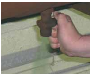
Compressed air contamination (condensate) being drained from a locomotive air receiver
